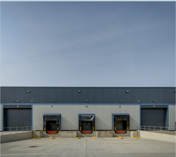
3 dock level doors & 3 level access doors
